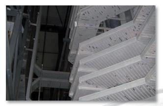
► Cable trays (perforated or solid sheet metal, insulator, wire) and cable ladders
