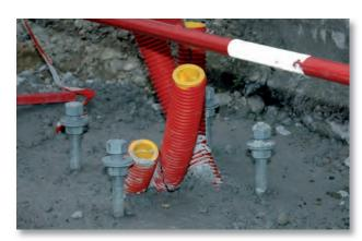
► Conduits (sheaths and cable protection tubes: CPT)
